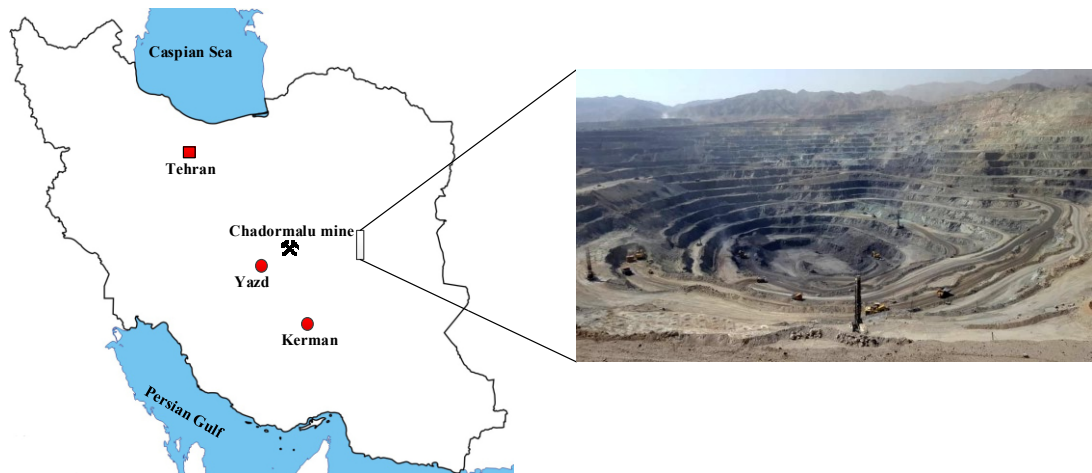
Figure 4. Location and a view of the Chadormalu iron ore mine of Iran
