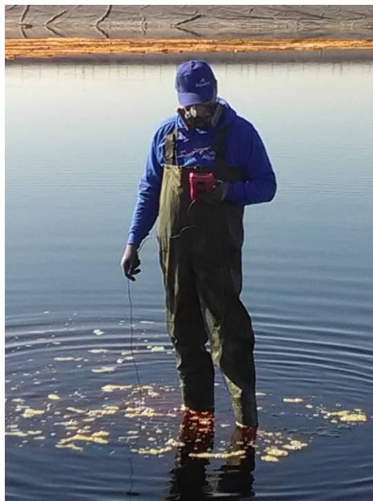
Figure 1. Technician measuring the tightness of the geomembrane insulation
