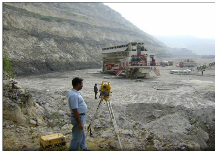
Figure 12. Establishment of baseline for orienting highwall miner for parallel web cutting using Total Station
